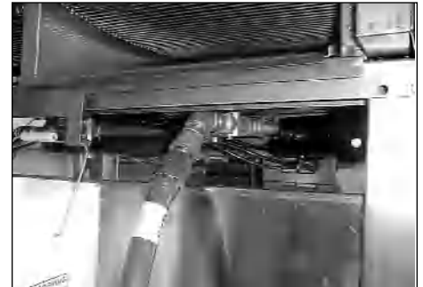
9015 Equipment Side Gas Connection
