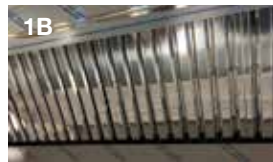
Grease-X-Tractor™ filters, first row of filters
