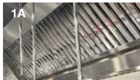
Grease-X-Tractor™ filters, first row of filters
