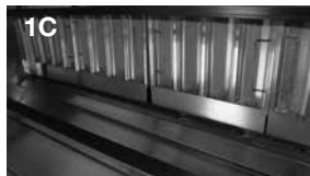
Grease Grabber™ filters, second row of filters
