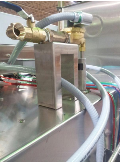
Showing hot water inlet, solenoid, and ASSE air gap
