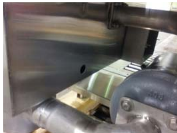
Showing 7/8" detergent probe hole behind pump motor
