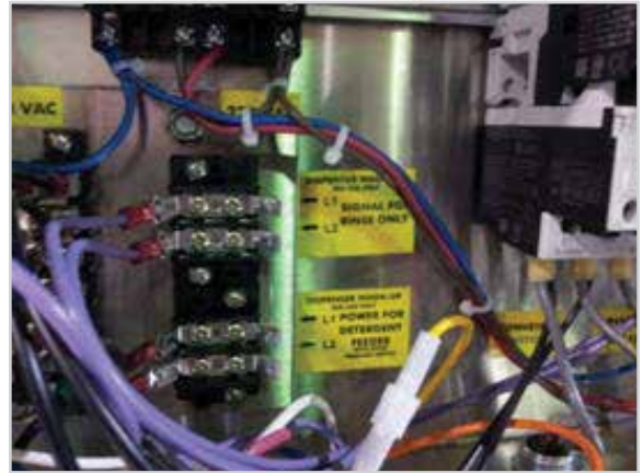
Dispenser signal connection terminals in control box
