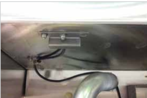
Sequence reed switch for wash tank
