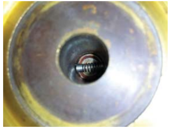
Failing to remove spring lodged in tube
