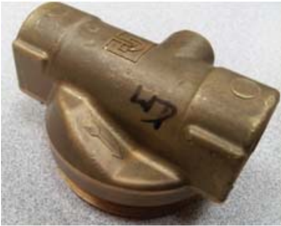
Installing valve wrong way, see arrow flow direction
