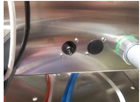
Chemical alarm barb adjusting screw *
