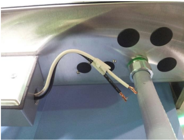
Showing control box, chemical pumps, prime switches
