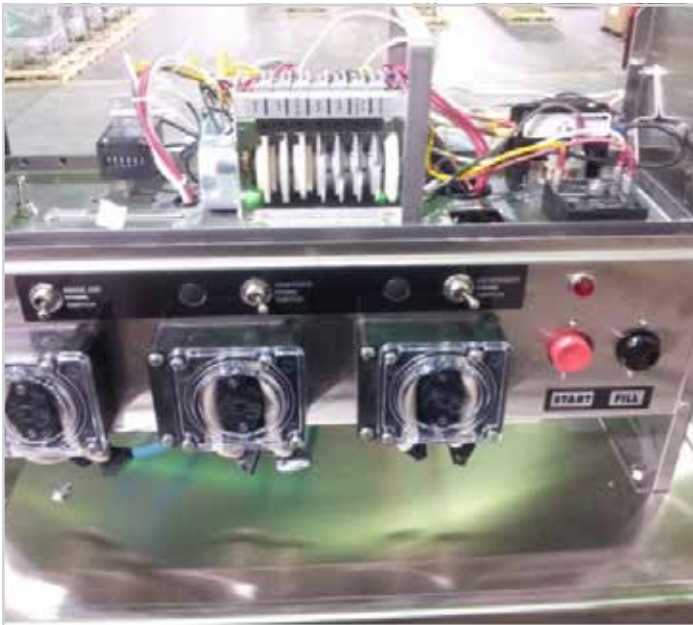
Showing control box, chemical pumps, prime switches
