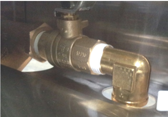
Drain hose connection to drain pipe
