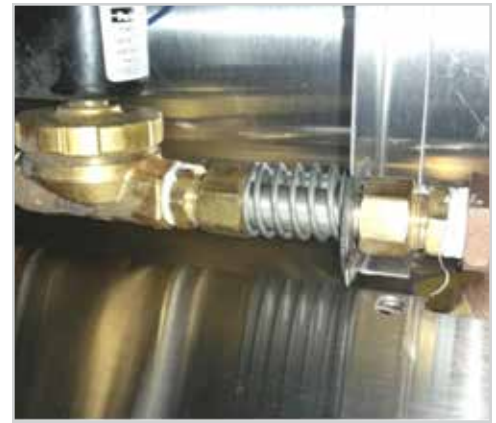
Compression connections for water solenoid
