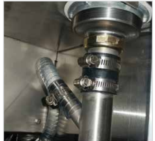
Drain hose connection to drain pipe
