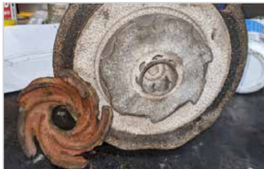
Impeller damaged from high acid solution
