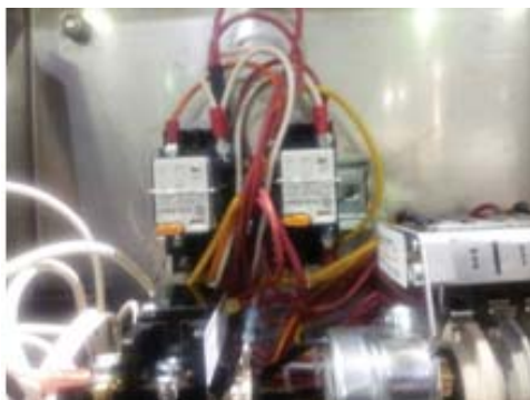
Left is Start Relay, right is Heater Relay Left is Drain Relay, right is Heater Contactor Optional buzzer for low chem. alarm
