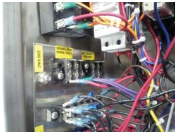
Showing dispenser signal connection terminals
