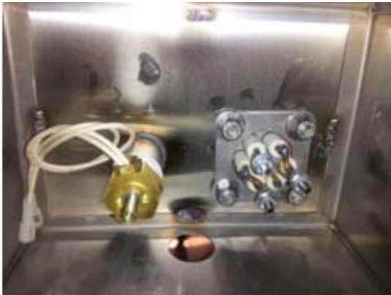
Showing thermostat and sustainer heater terminals*
