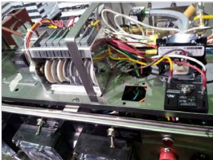
Showing control tray installed in normal position
