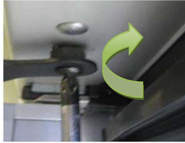
Tighten Hold-Open Screw
