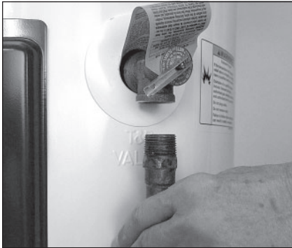
Figure 11 - Removing the T&P Relief Valve discharge pipe.
