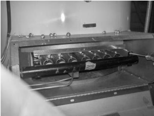
Step 7: Remove manifold bracket screws
