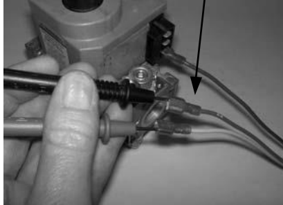
Check across "MV/PV" & "PV" Wire leads to gas valve
