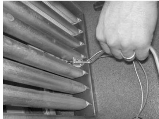
Step 16: Slide pilot assembly to back of burner rack
