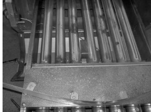
Step 14: Slide out burner assembly
