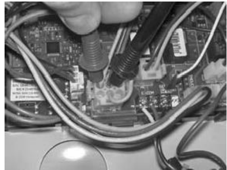
Checking MV & MV/PV control plug pins to gas valve for 24 volts output during heating cycle (pilot must be lit with no sparking).
