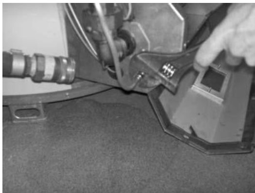
Step 3: Disconnect Pilot Fitting from Burner Box
