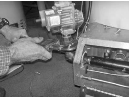
Step 5: Disconnect and Remove Gas Valve
