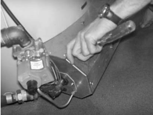
Step 1: Remove burner box cover screws
