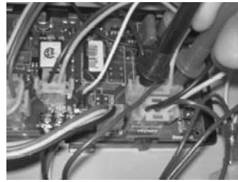
Checking line voltage to board. Pins to black and white wires.
