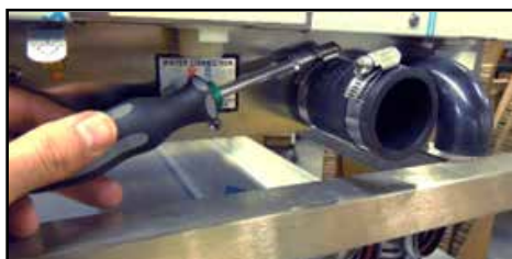
Tightening the hose clamp for the drain coupler
