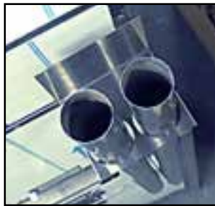
Slide the bracket down from the top
