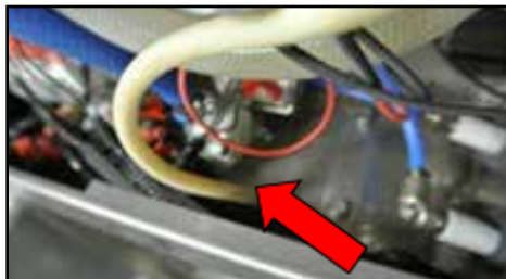
Installed grommet in the hole.
