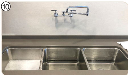
10. Prepare one-gallon (3.8 liter) of sanitizing solution with at least 100 ppm of available chlorine in 120°F (48.9°C) water. Clean all parts in compartment sink.
