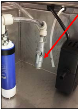
Fig. 3 Priming valve in OPEN position
