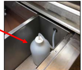
Fig. 3 Dry box with pH dosing bottle
