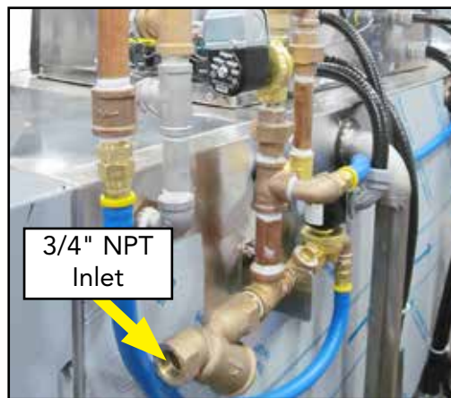
Fig. 5 - No booster may not require a PRV.
