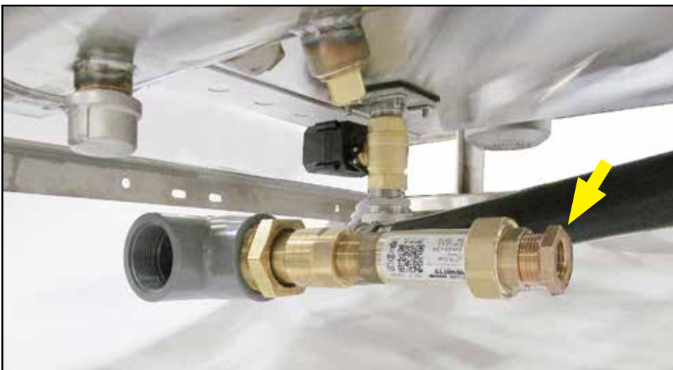
Fig. 6 - Mechanical DWT valve.
