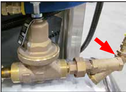
Fig. 8 - Standard and Heat Recovery hot water connection
