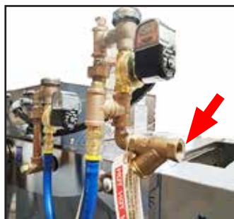
Fig. 9 - Hot water connection no internal booster
