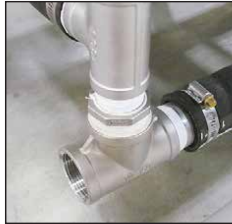
Fig.16 - Single tank with prewash drain connection
