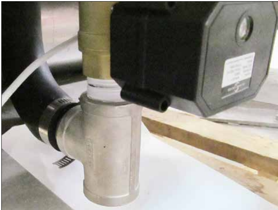
Fig. 7 - 1" NPT electric drain valve connection
