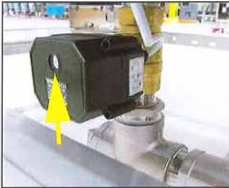
Type 1 - Without adjusting knob
