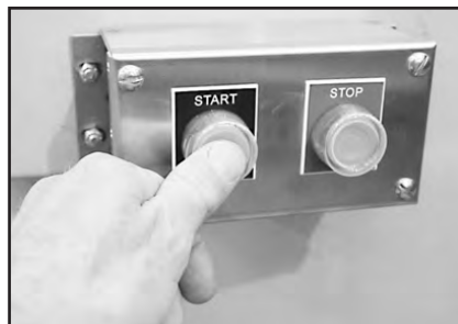
Start/Stop Station ON.
