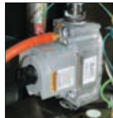
7. Gas Valve (showing hose for pressure tap)
