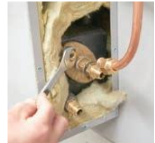
Fig. 6.4 Loosen the oval flange.
