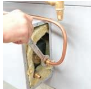
Fig. 6.3 Loosen the water input tube.
