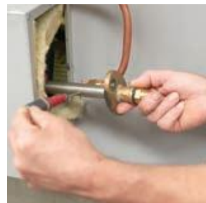
Fig. 6.5 Remove the filter and clean the limestone from all of the openings.
