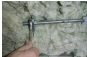
Fig. 2.4 Tighten springs.
