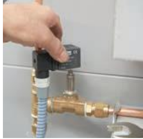
Fig. 7.2 Remove the coil.
