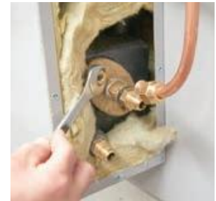
Fig. 6.4 Loosen the oval flange.
