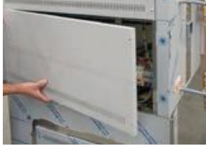
Fig. 4.1 Loosen the screws on the right panel.
