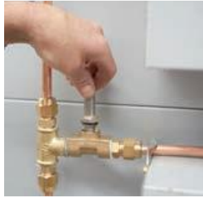
Fig. 7.4 Carefully remove the piston.
