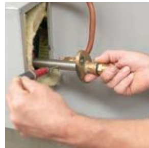
Fig. 6.5 Remove the filter and clean the limestone from all of the openings.
