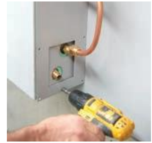
Fig. 6.2 Loosen the back panel.
