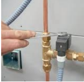
Fig. 7.1 Loosen the nut (remove it).
