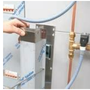
Fig. 6.1 Loosen the back steam output.
