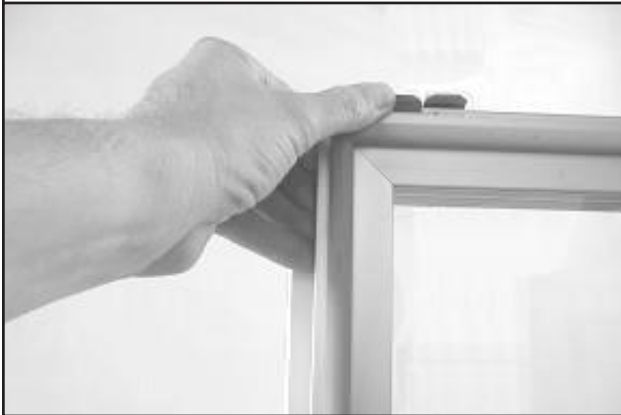
1. To open the windows for cleaning, unlatch the top clip.
