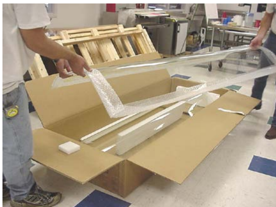
Step 5. Remove curved glass from box. Remove protective wrapping from glass.
