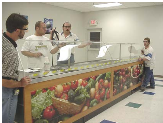
Step 11. Slide second piece of glass next To first piece of glass to snugly fit against U-channel in center.
