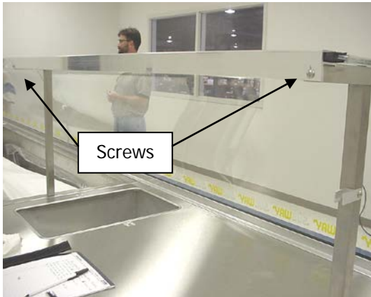
Step 15. Secure upper extrusion with screws and nuts. Rubber gaskets are supplied long. Trim excess from ends.
