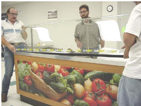
Step 7. Place glass with rubber gasket into bottom extrusion. Align edges of glass and extrusion. Put vinyl U-channel over edge of glass at center of counter.
