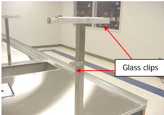
Step 3. Place leg with two glass clips over leg block on Hot Food Unit. Secure with screws.
