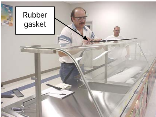
Step 13. Place rubber gasket over top edge of both pieces of glass.
