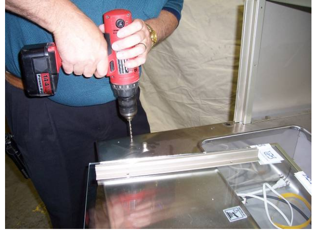
27) Using 5/32" bit, drill the two holes.
