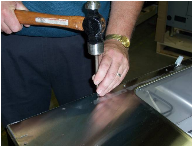
12) Center punch the location where each hole is to be drilled.
