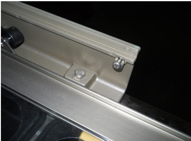
15) Add glass clips from old pylon to new pylon
