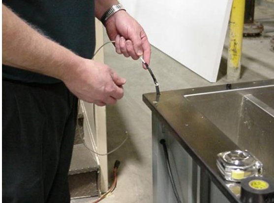
13) Pull Fish wire up through top hole with Electrical Wire attached.
