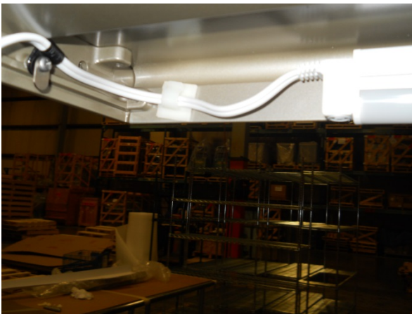
27) Push cord thru light clip on top and plug light cord into light fixture
