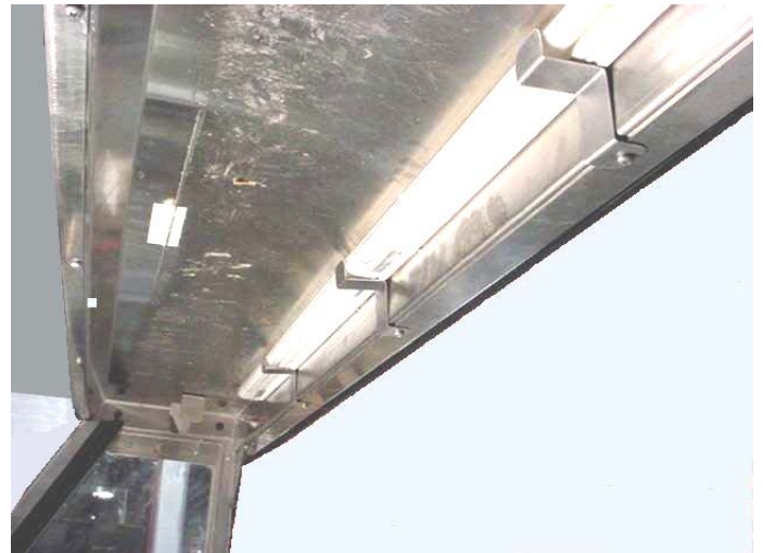
Fully installed and plugged in with lights on.
