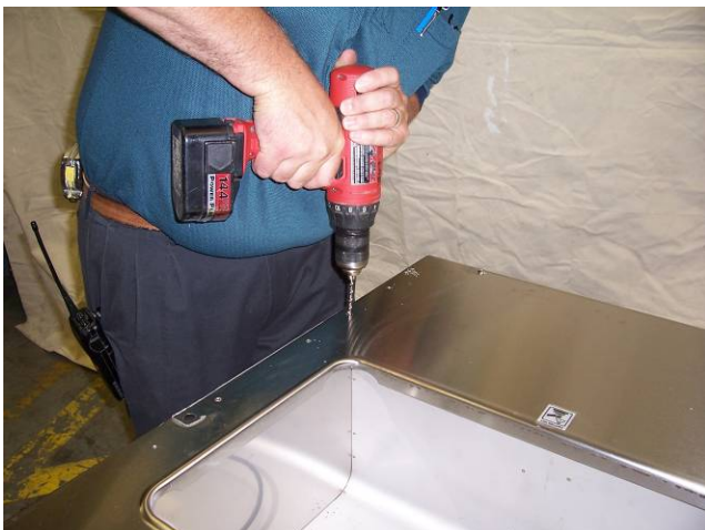
14) Using a 5/32" bit, drill the 6 holes that will be used to bolt down the new Painted Aluminum Day Cover.
