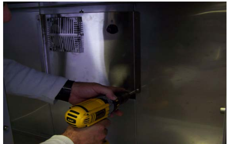
Re-Install the Fan Motor Cover using the (4) existing screws. Note: Be careful to align the fan blade to the center of the ring on the fan cover. It must have the proper clearances from the ring to operate properly.
