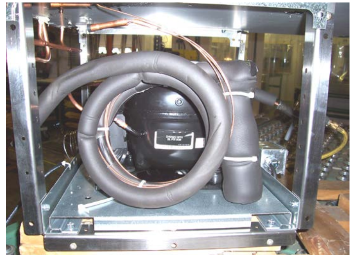
22. Dress any remaining ties and ensure the courtesy loop is recoiled correctly as shown in the figure.
