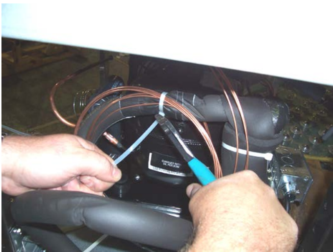
19. Beginning with the twelve o'clock position, secure the capillary tubing, and dress off the excess tie.
