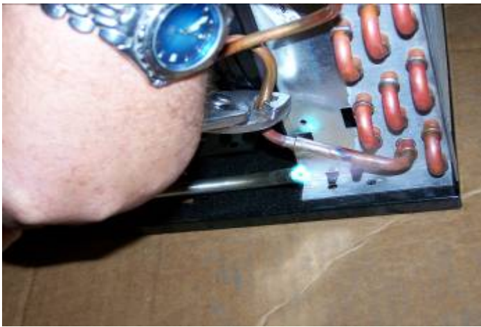
8. Unsweat the liquid line assembly at the condenser outlet.
