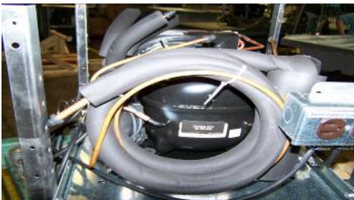
12. Slide the condensing unit back into place and bolt back down to cage.
