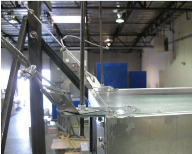
FIGURE 5 – OVERLAPPED FLAT, 90° AND 45° BRACKETS
