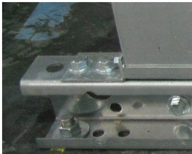
FIGURE 10 – BOLT AT EACH BASE-RAIL CORNER
