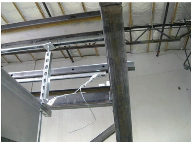
FIGURE 3 – LATERAL SUPPORT COMPONENTS FOR HDD 08-20
