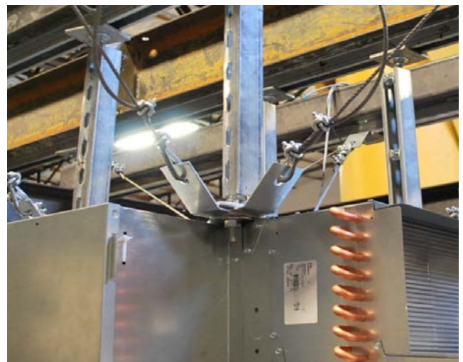
FIGURE 7 – OVERLAPPED FLAT AND 45° BRACKETS
