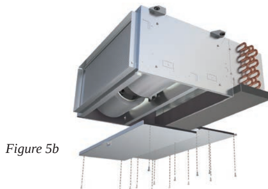
Figure 5a-5b: Bottom panel removal
