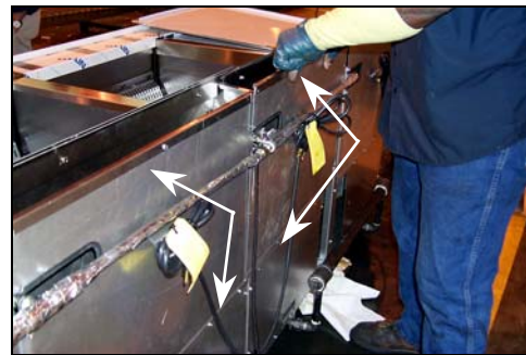
Figure 2. Removing cabinet backs to access connection points.
