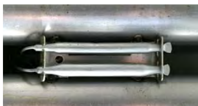
Typical high-limit/sensor probe locations and mounting hardware.
