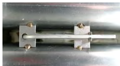
Typical high-limit/sensor probe locations and mounting hardware.
