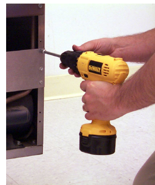
Removing gas manifold shield.
