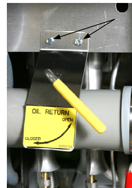
Oil-return handle bracket and screws.
