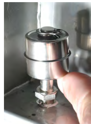
High-level float switch
