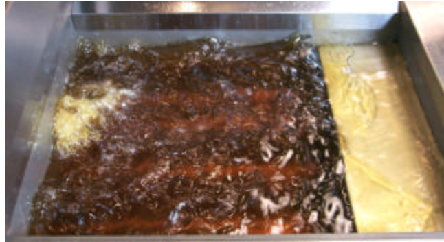
Bubbling oil indicates air is being pumped through the oil return lines.
