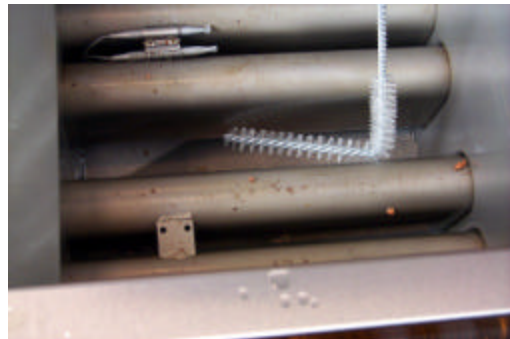
Cleaning fry-vessel tubes and bottom with "L-shaped" brush.
