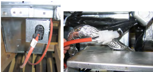
Figure 6: Attach the two-pin white connectors and plug the black connector into the utility box as shown. * Note the position of the black connection may differ from photo.
