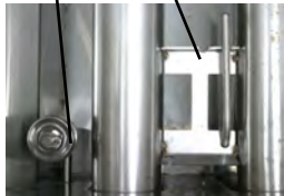
Low-water float switch, Temperature probe
