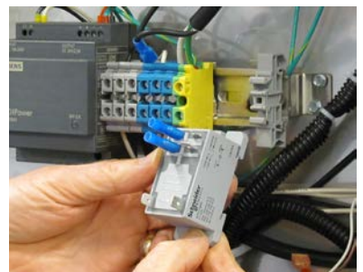
Push up on bottom of relay, angle top off upper rail flange to release.
