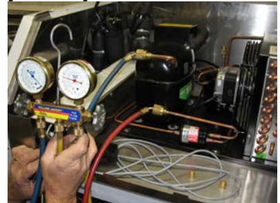
Check Discharge and Suction Valve pressures using a manifold refrigeration gauge.
