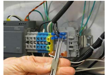
Remove wire terminals from Control Relay.
