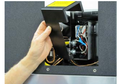
Remove screw & slide up/off relay box cover.
