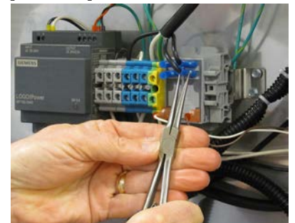
Disconnect three condenser power cord wires from DIN-rail mounted terminal block & relay.
