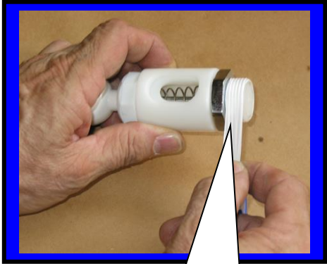
Faucet Assembly C6513 . Teflon Tape added before installation
