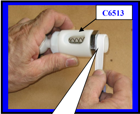
Applying Teflon Tape to Faucet Body before installation
