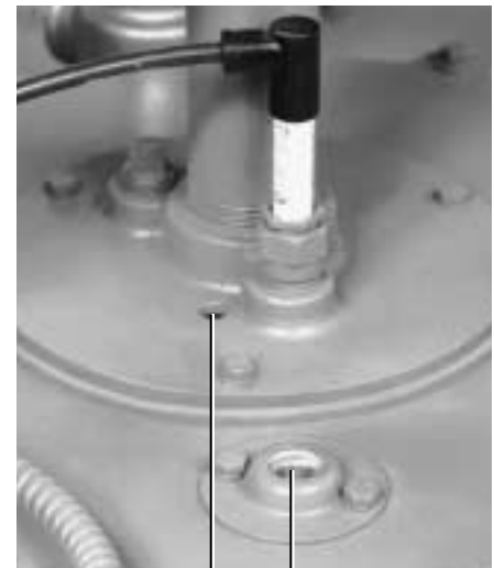
Burner Viewing Port Blast Tube Viewing Port
