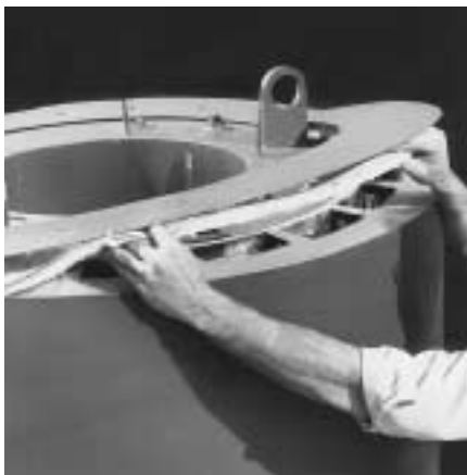
Remove burner and flue cover plate
