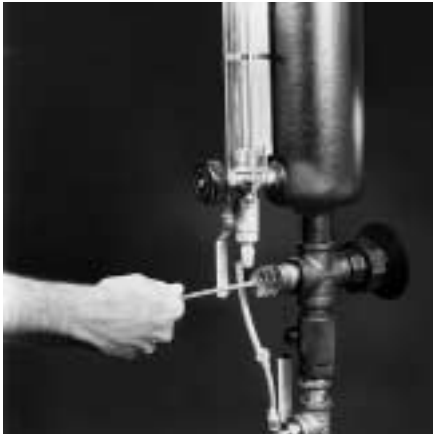
Remove plug at cross section; clean nipple to boiler.
