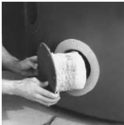
Removing clean out plugs.
