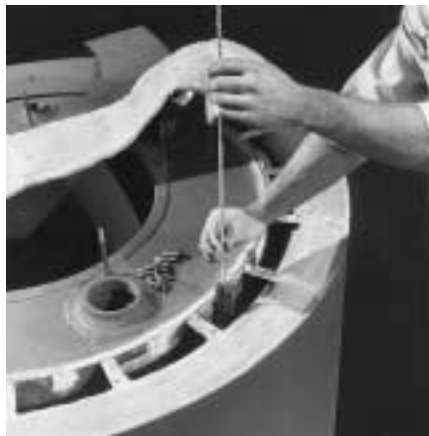
Wire brushing the flue passages.
