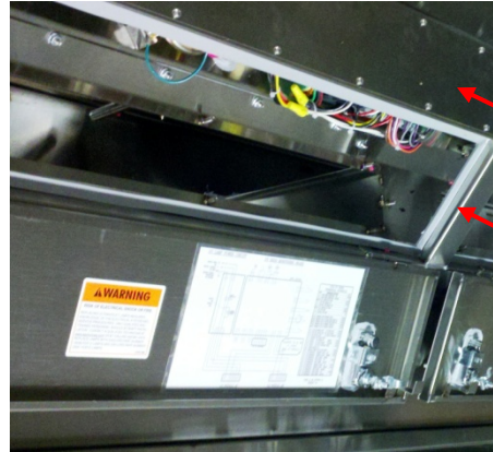
Figure 6-31-1 Main Electrical Raceway Access Panel
