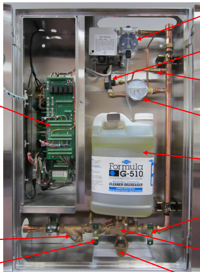
Figure 4-41-1 Typical Main Control Cabinet (Sub Panel is the Same Except Without Control Compartment
