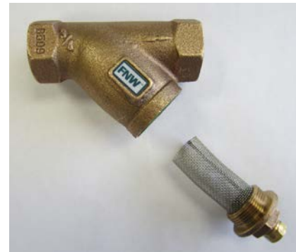
Figure 4-48-2 Line Strainer With Screen Removed
